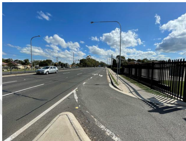
Figure 3.4 – Cumberland Highway (looking south)
