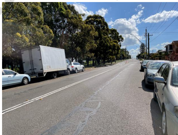
Figure 3.6 – Brenan Street (looking west)
